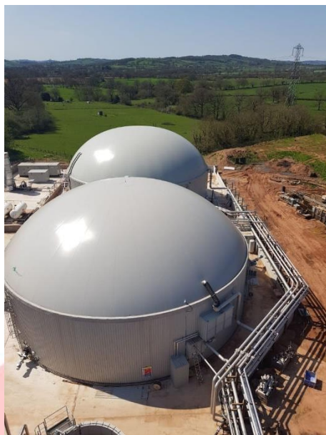
Copyright Biogest - Biomethan plant Willand, Royaume-Uni
